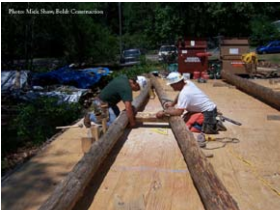
Workers from Bachmann Construction install the webs of the truss
