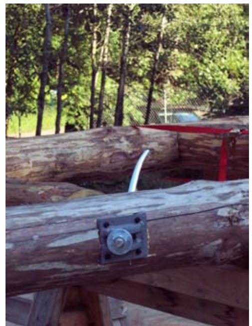
Threaded steel pipe spans the area between webs, strengthening the truss
