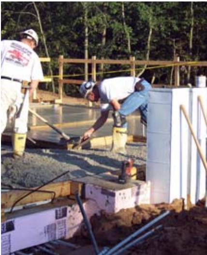
Concrete is carefully smoothed over the plastic tube system
