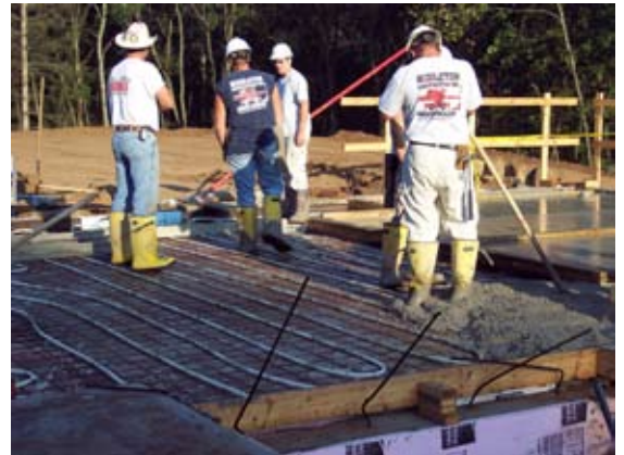
Workers pour concrete over tubing to form floor slabs
