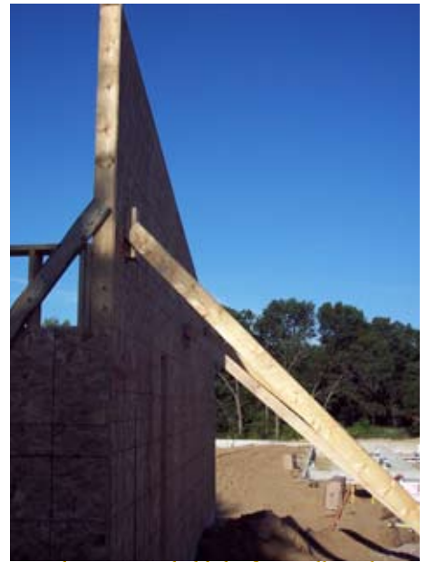
Wooden supports hold the first wall in place
