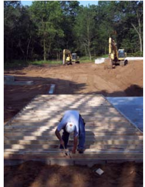
Worker from Bachmann Construction nails wall studs in place.
