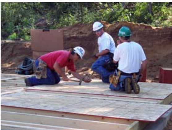
Workers attach plywood sheets to wall studs
