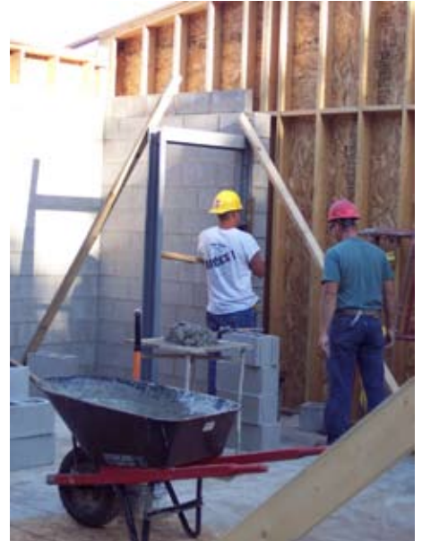
Workers lay cinderblocks for fire-proof storage closets.
