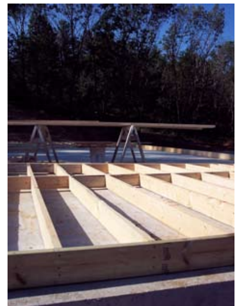
The wall is ready for a layer of plywood
