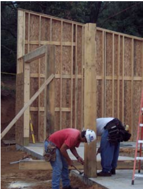
Workers anchor Leopold pine beams that will frame the garage doors
