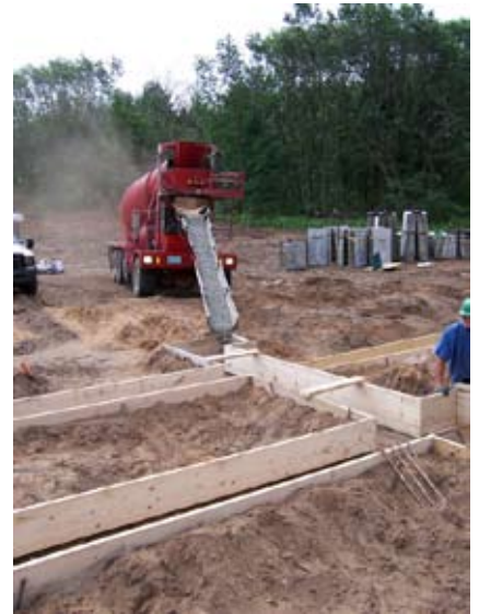
Concrete is poured into the wooden forms
