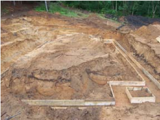
Wooden forms will hold the foundation footers
