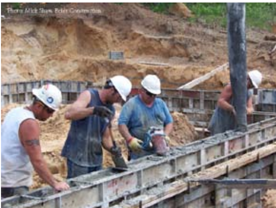
The crew pours concrete into aluminum wall forms
