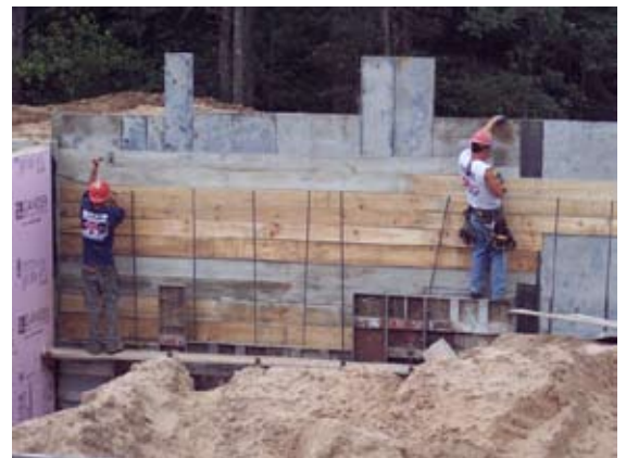
Leopold pine boards create a textured surface in the concrete
