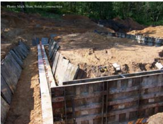
Aluminum forms mark where foundation walls will be
