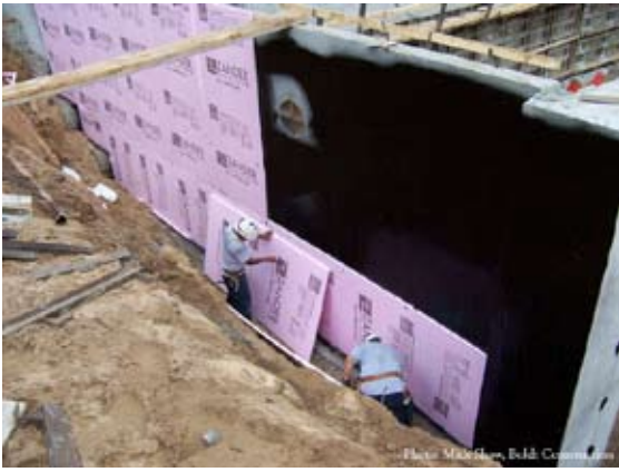
Finished wall is sprayed with waterproofing and covered with insulation
