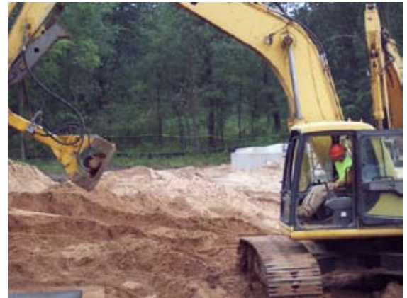
Backhoe creates compacted soil surface for pouring floor
