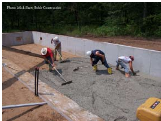
Crew smooths concrete into floor
